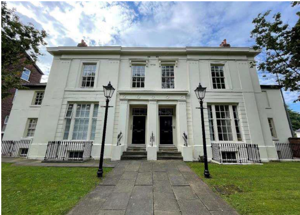
View of existing Grade II listed building 466 – 468 Moss Lane East as viewed from Moss Lane East
